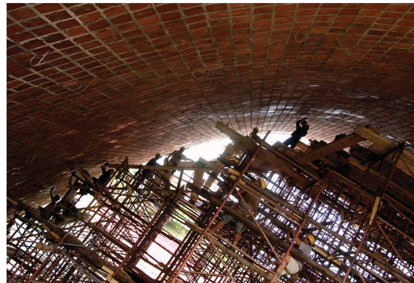
Building works of the new vault, Summer Theatre "Ramón Collazo". December 19, 2006. (Photo number: 20073FMCMA.CMDF.IMM.UY - Autor: Carlos Contrera/CdF)
